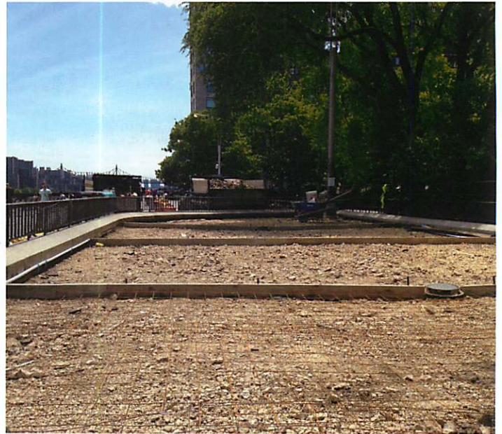
The SDR before the new surface is poured.
