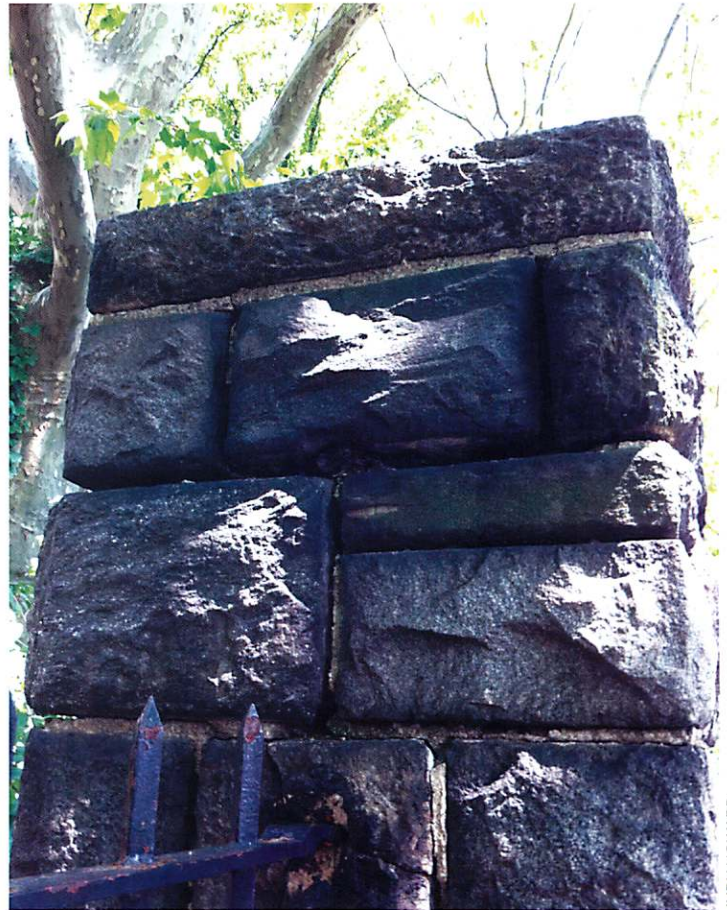
Carl Schurz Park stonework ready for repair.
