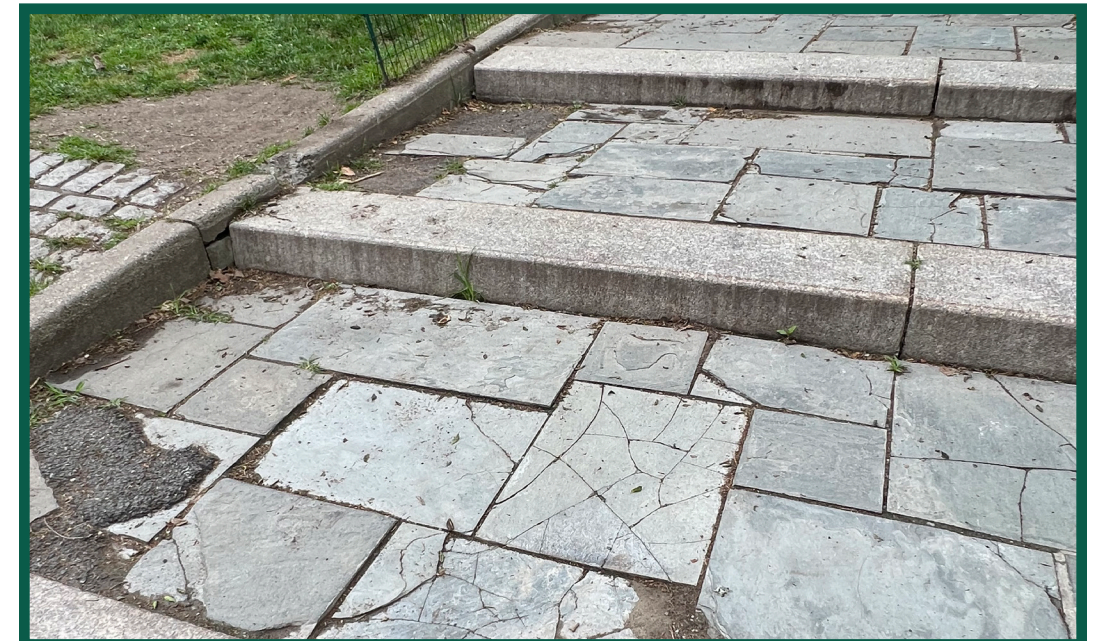
Top, the restored staircase. Above, before.
